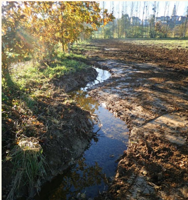
Water way rewinding work
