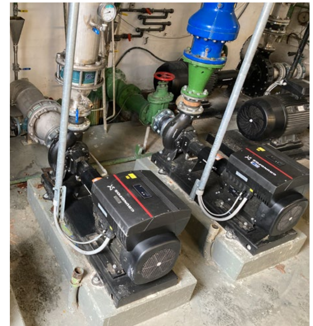
Replacement of water supply pumps with high efficiency pumps at our Lindau, Germany facility
